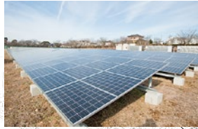
太陽光発電設備 Photovoltaic Facility
