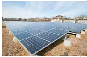
太陽光発電設備 Photovoltaic Facility
