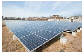
太陽光発電設備 Photovoltaic Facility
