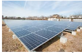
太陽光発電設備 Photovoltaic Facility
