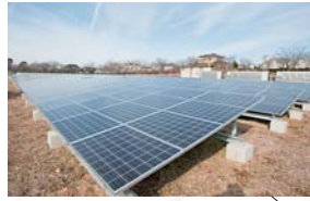
太陽光発電設備 Photovoltaic Facility
